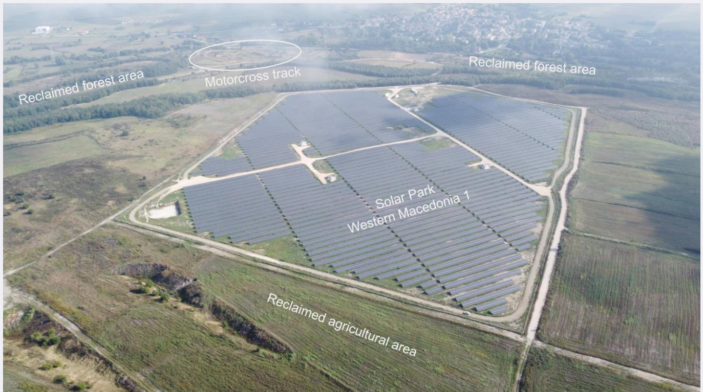
Land restoration and a 15 MW solar PV park near Ptolemais at the West Macedonia Lignite Centre – part of the 550 MW Kozani solar project
