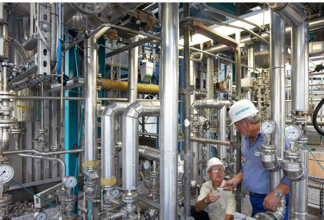
6 — Post-combustion carbon capture installation at German power plant Staudinger
