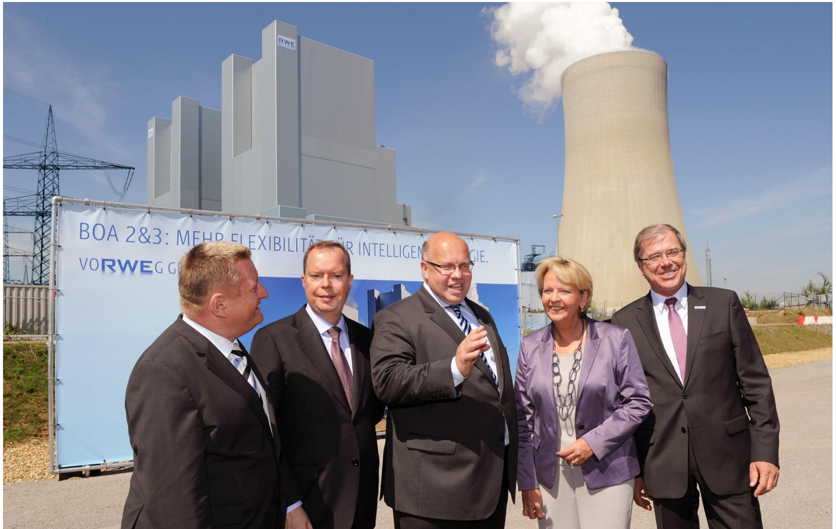
RWE BoA 2 & 3 lignite-fired power plants at Neurath in Germany
